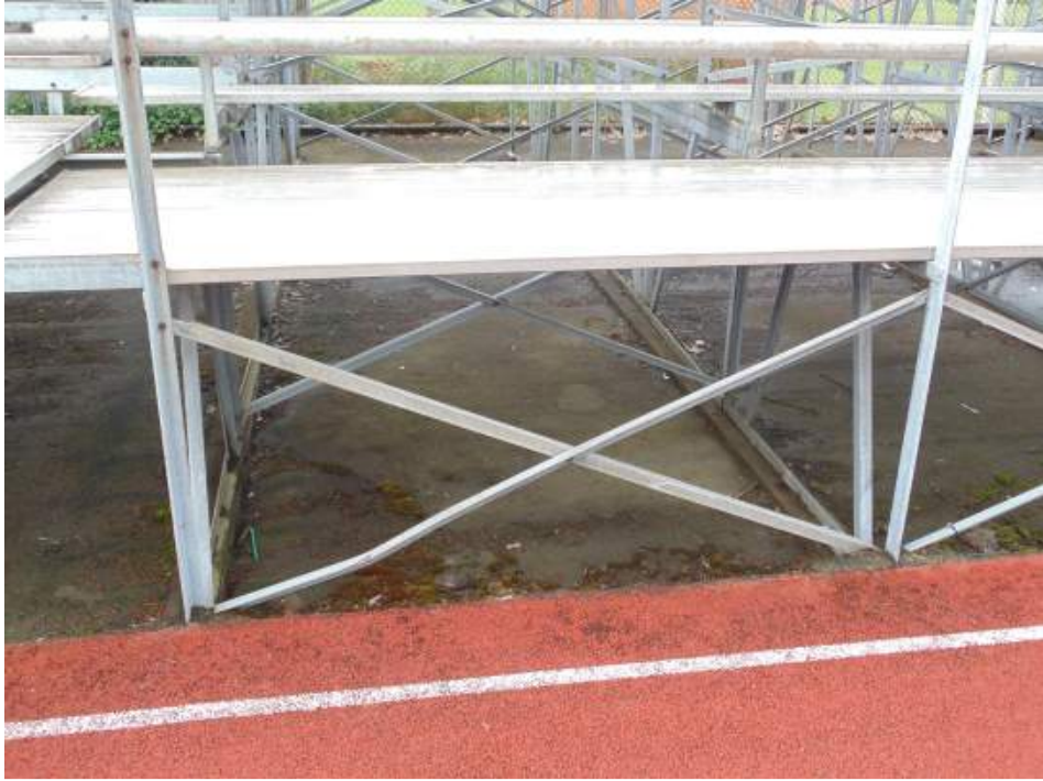
FIGURE S1: BENT CROSS FRAME ANGLE
