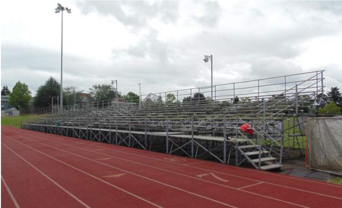
North View of Bleacher
