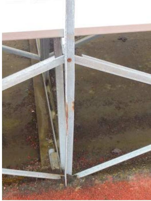
FIGURE S3B: DENTED ANGLE
