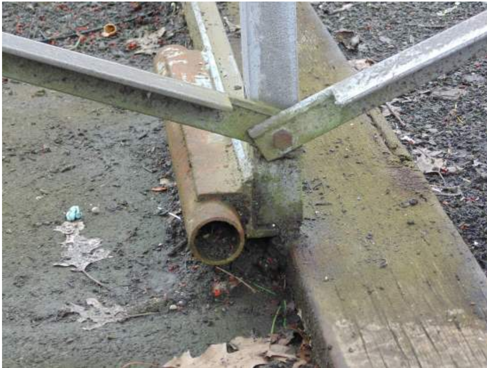
FIGURE W2: BASE ANGLE HANGING OFF SUPPROTING WOOD
