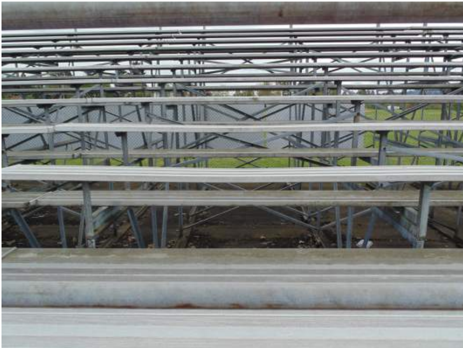
FIGURE S9: TYP. MINOR BENDING IN SEATS
