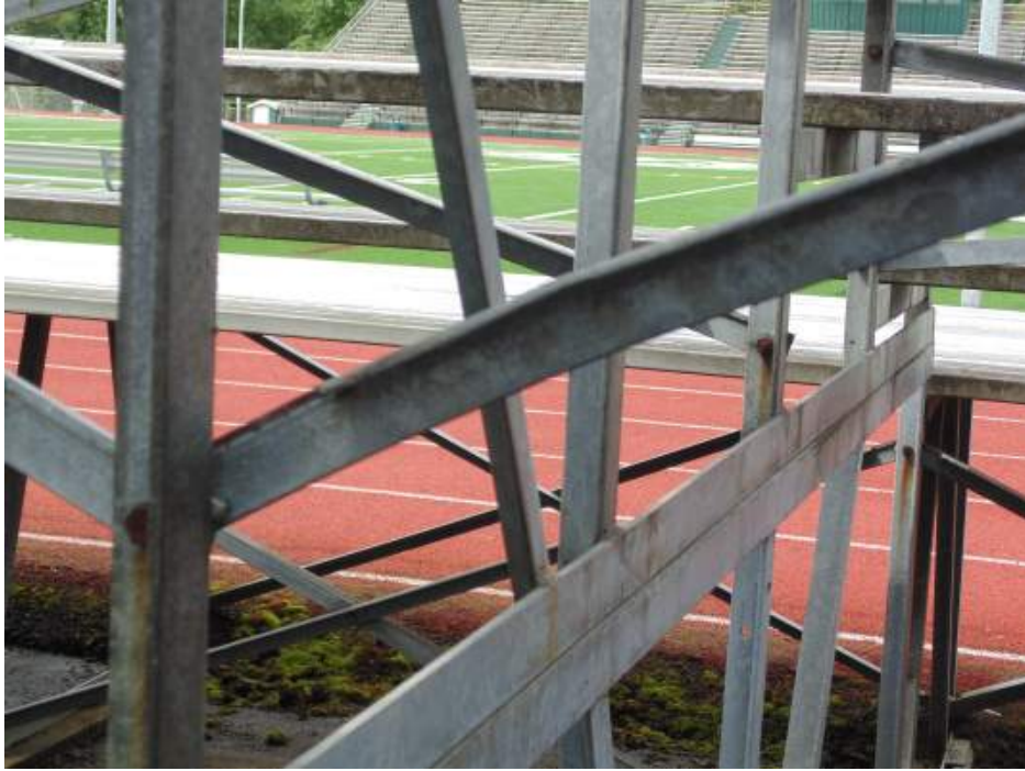
FIGURE S4: BENT ANGLE
