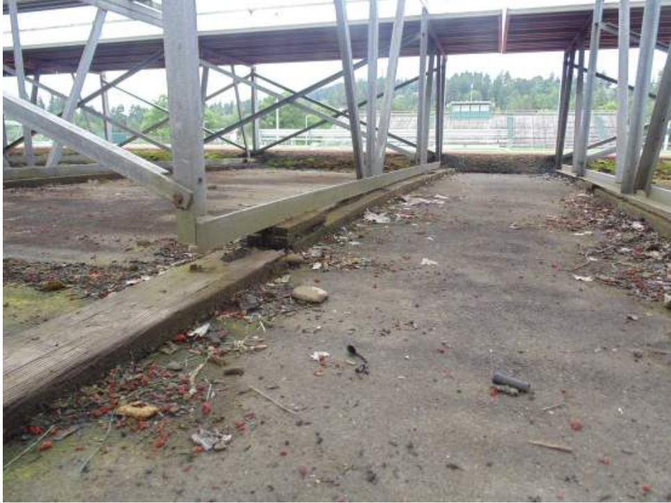
FIGURE W3: BASE ANGLE FLOATING AT POINT OF SUPPORT
