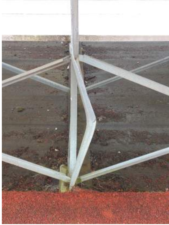
FIGURE S2B: BENT ANGLE
