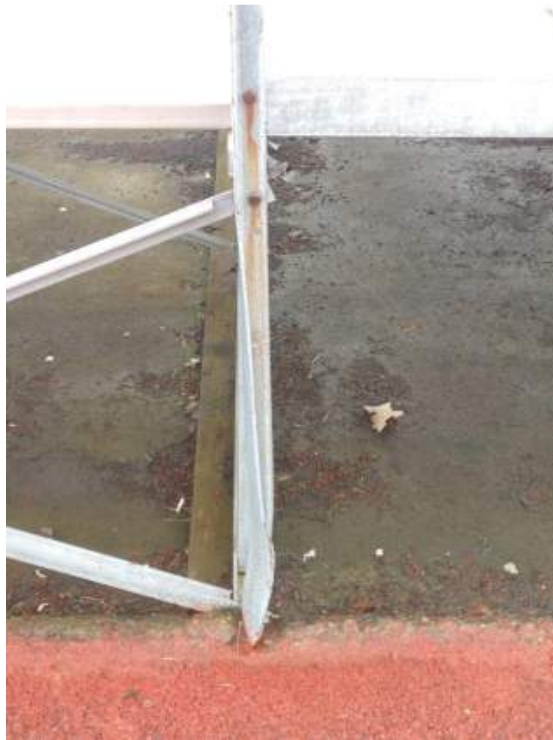
FIGURE S2A: BENT ANGLE
