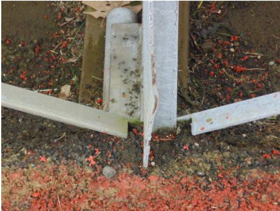
FIGURE S3C: DENTED ANGLE
