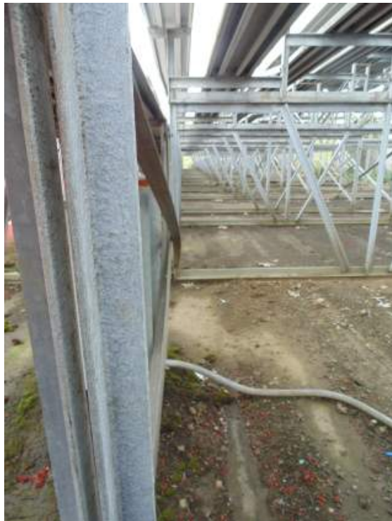
FIGURE S5: WARPED ANGLE
